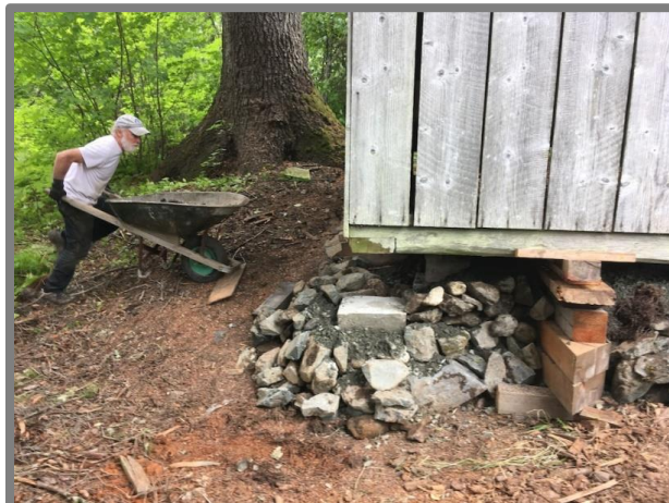
Volunteer, Tim McDonough working on the Anway woodshed restoration—summer, 2018.
